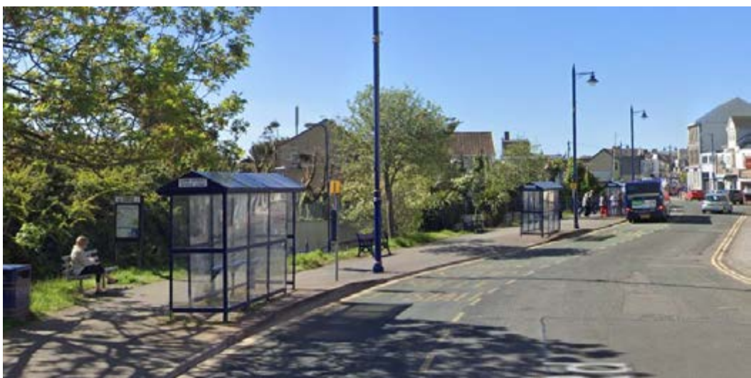
Photograph 3.3 Existing Porthcawl Bus Station
