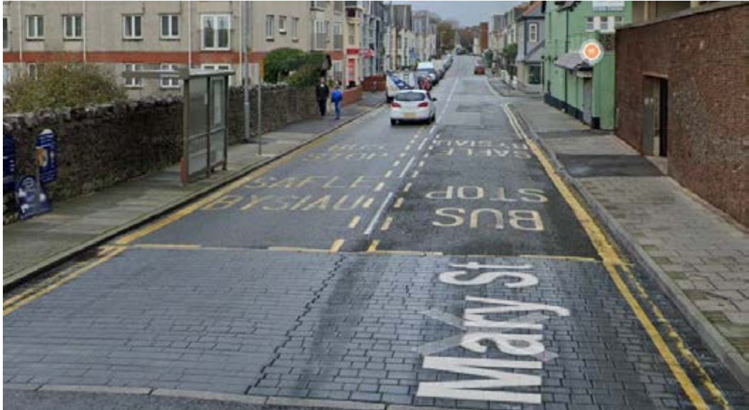
Photograph 3.2 Mary Street north & southbound bus stop
