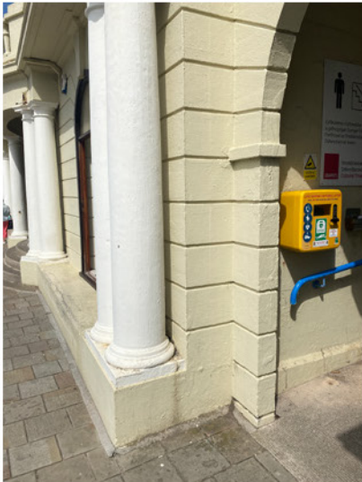
Detail of front façade
