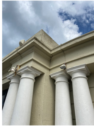
Detail of front façade
