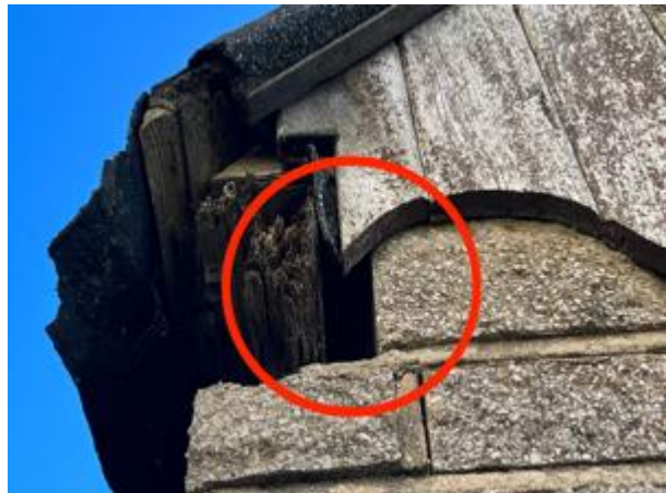
Photo 28: Gap Present in Roof, Detached Porch, Cricked
