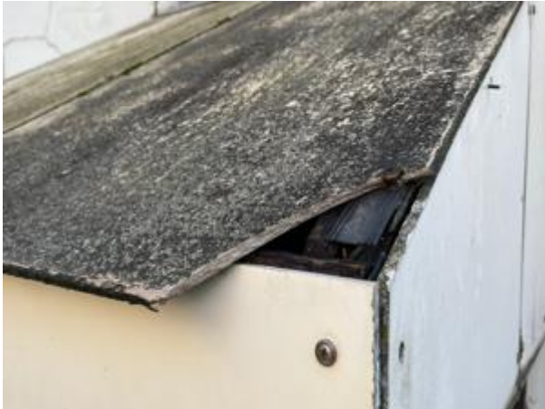
Photo 11: Broken Tile Present on Roof, Western Elevation
