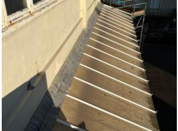
Photo 10: Lead Flashing Removed from Monopitched Roof, Western Elevation
