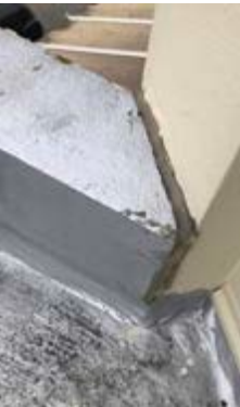
Poorly Detailed Junctions Manyllder Gwael i Gydiadau
