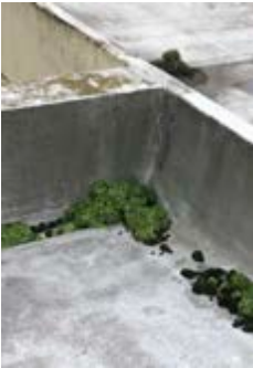
Poor Falls to Flat Roofs Rhaeadru Gwael i Doeau Fflat
