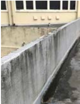
Ingress and Weathering to Parapets Mynediad a Hindreulio i Barapetau
