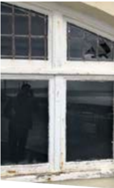
Decay to Clerestory Window Frames Pydredd i Fframiau Ffenestri Llofft Olau
